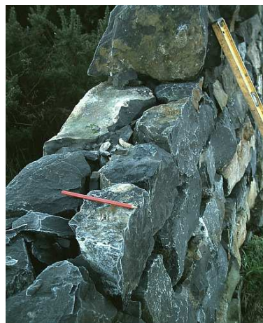
Fig.33. Stones traced on edge. It can be seen that length of pencil into wall is less than if it was held up the face.
