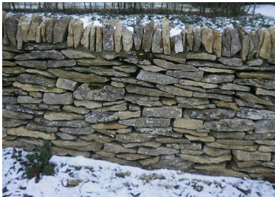
Fig Fig.17. Left and right, sections of same oolitic limestone wall built by different contractors
