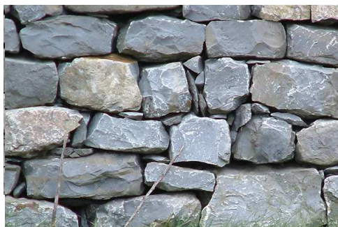
Fig.30. Front pinning
