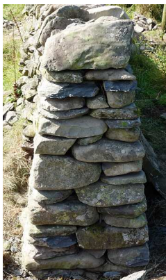
Fig.55. End and side view of reasonable broken tie wall end.
