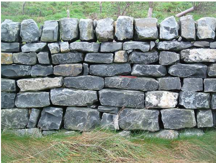
Fig.8. Excessive grouping of traced stones
