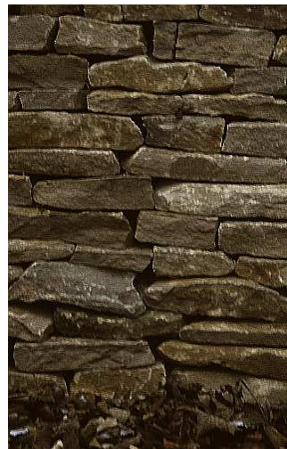
Fig.28. (l to r) Zipped joints in (l to r), glacial field stone, sandstone, oolitic limestone
