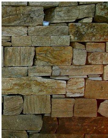
Fig.32. An excess of plates in sawn sandstone wall
