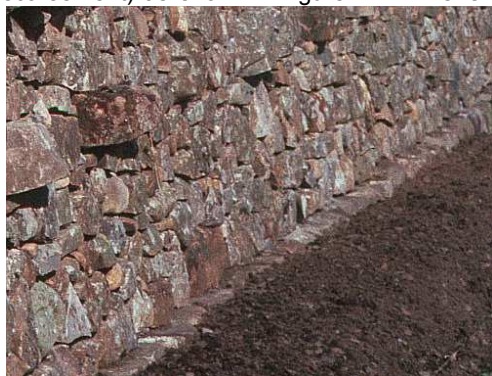
Fig.42. Wall with a scarcement
