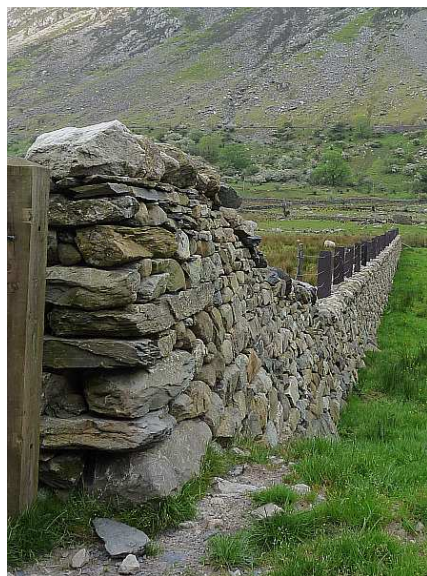
Fig.39. Good line and batter
