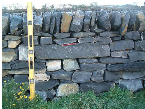
Fig.7. Excessively traced stone (1.2m level)
