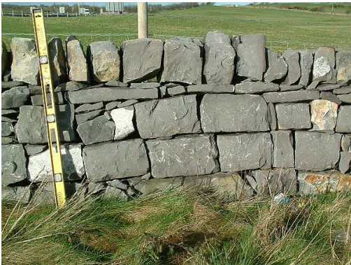
Fig.4. Oversized stones high in wall, carboniferous limestone
