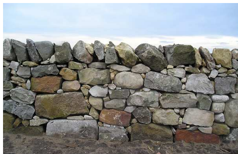
Fig.31. Badly built pinned wall Brora, Sutherland
