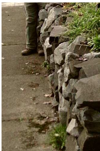
Fig.38. A severe bulge is a fault in both line and batter
