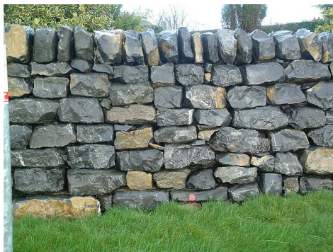
Fig.29. Stacking in regular shaped limestone
