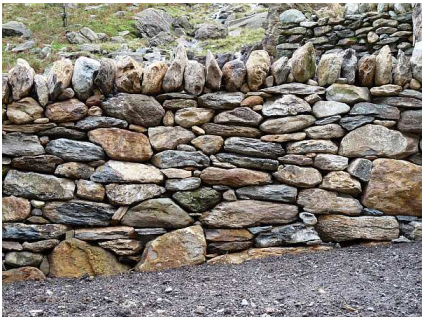
Fig.9. Face view and inside view of an extremely badly traced wall
