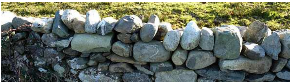
Fig.50. Poorly structured and poorly fitted rubble coping
