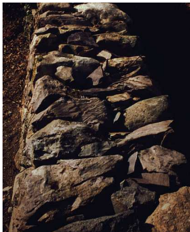
Fig.49. Good 'double rubble' coping left, poor rubble coping right.
