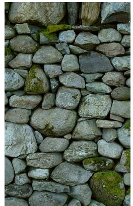
Fig.26. Diagonal running joint (centre), in glacial fieldstone wall
