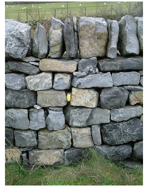
Fig.24. Running joint in regular limestone
