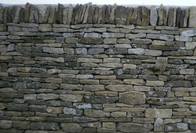
Fig Fig.17. Left and right, sections of same oolitic limestone wall built by different contractors
