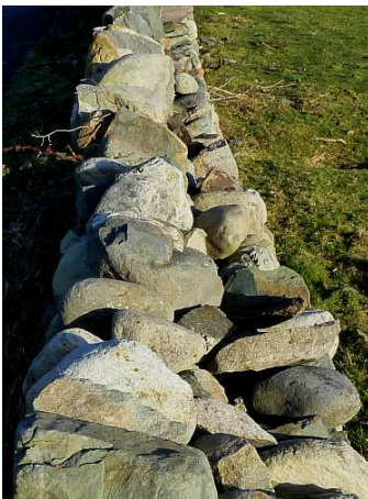
Fig.49. Good 'double rubble' coping left, poor rubble coping right.
