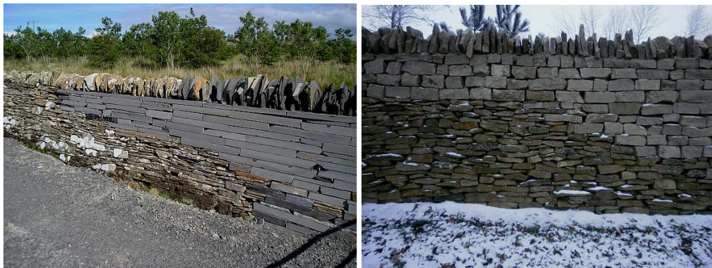
Fig.1. Inappropriate stone used in repairs Caithness (left), Cotswolds (right)
