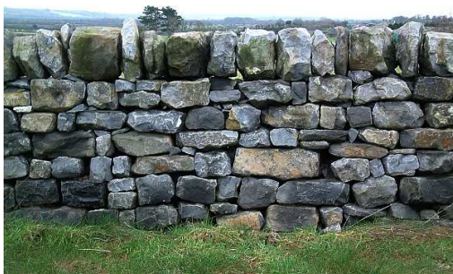
Fig.12. 2 sections of wall from very similar carboniferous limestone, showing a tight face (left) and relatively slack face (right)
