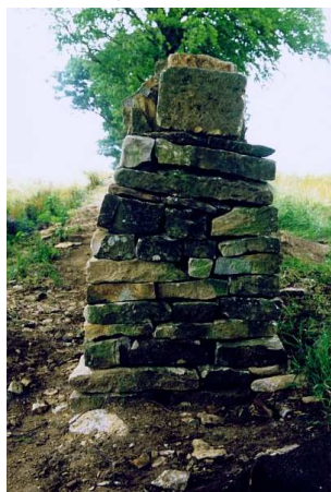
Fig.54. Poorly constructed "broken-tie" wall end
