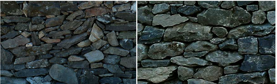
Fig.36. Adjacent garden walls of same stone type, incorrectly set to level in left photo
