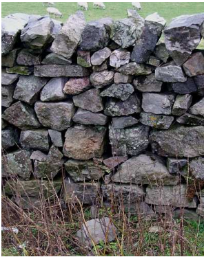
Fig.23. Running joint in irregular sandstone
