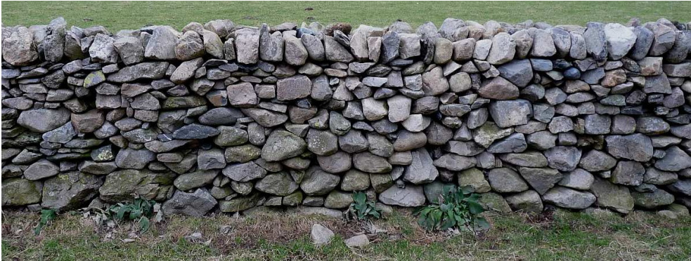
Fig.16. Above and below 2 sides of same field walled with glacial stone from field clearance. The top wall is built by trainees the lower wall by a Master Craftsman
