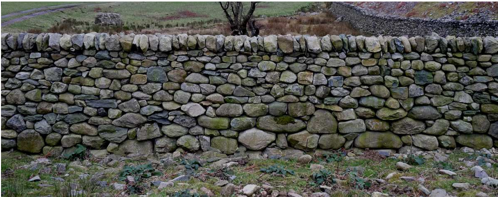
Fig.16. Above and below 2 sides of same field walled with glacial stone from field clearance. The top wall is built by trainees the lower wall by a Master Craftsman
