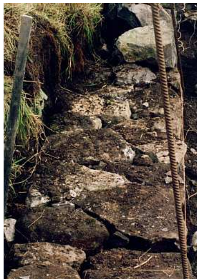
Fig.41. Flat/level, interlocking footing
