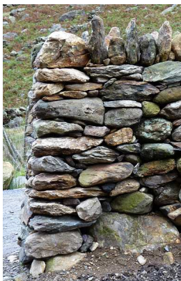
Fig.56. End and side view of badly tied 'broken-tie' end with insufficient batter.
