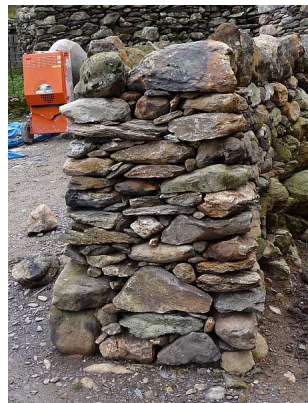
Fig.56. End and side view of badly tied 'broken-tie' end with insufficient batter.
