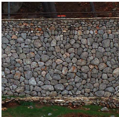
Fig.37. Polygonal wall, Mallorca
