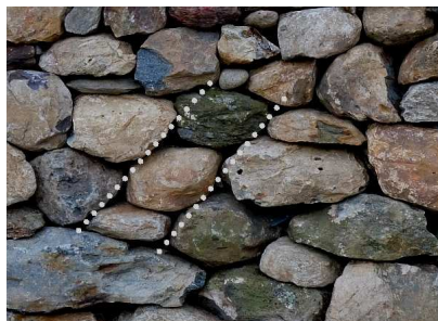
Fig.27. “Phantom” diagonal joints
