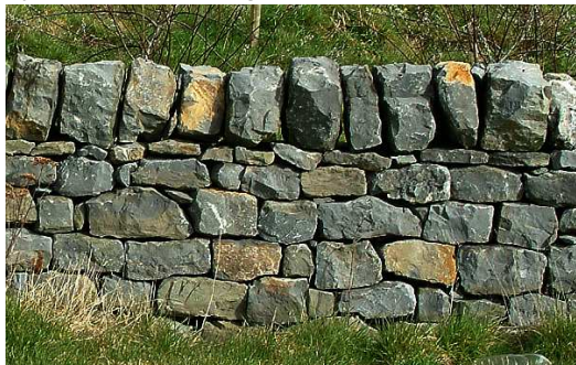
Fig.12. 2 sections of wall from very similar carboniferous limestone, showing a tight face (left) and relatively slack face (right)
