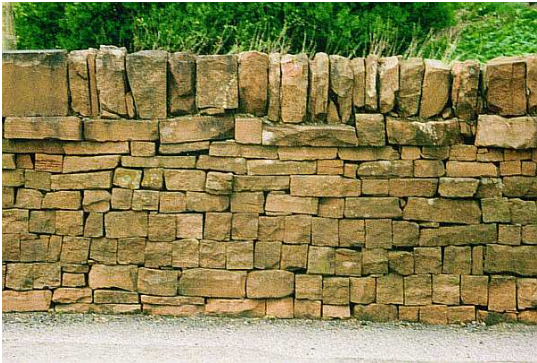
Fig.22. Excess of double joints in Permian red sandstone
