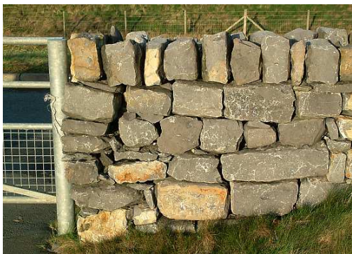
Fig.52. Poorly tied wall end with a lack of runners/stretchers.
