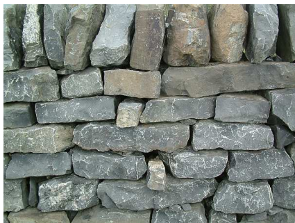
Fig.18. “Letterboxes” and loose stones
