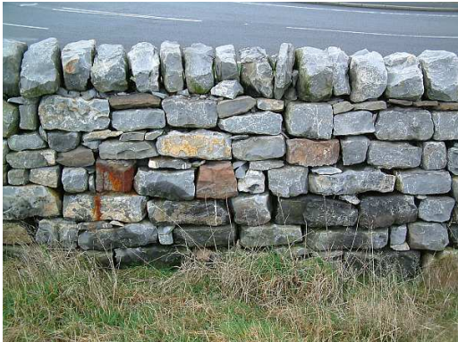
Fig.20. Wall riddled with “plumb” joints
