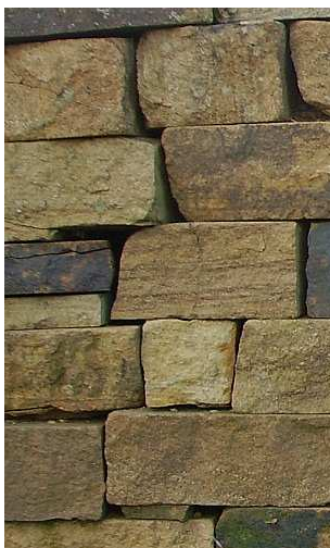
Fig.28. (l to r) Zipped joints in (l to r), glacial field stone, sandstone, oolitic limestone
