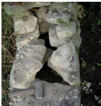
Fig.40. Voids were left as wall was built.
