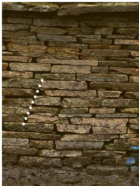
Fig.25. Diagonal running joint (left of centre), in sandstone wall
