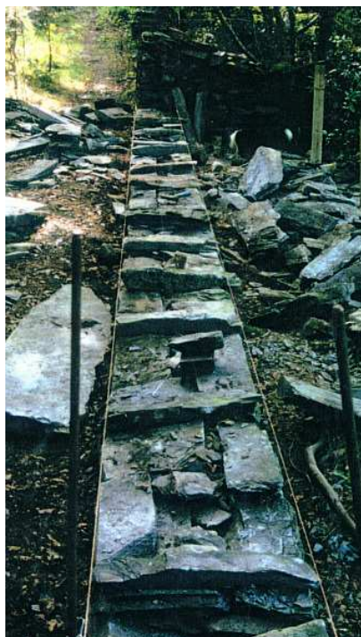
Fig.45. Regularly spaced flush throughs on a slate wall
