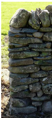
Fig.55. End and side view of reasonable broken tie wall end.
