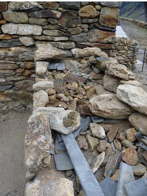
Fig.9. Face view and inside view of an extremely badly traced wall
