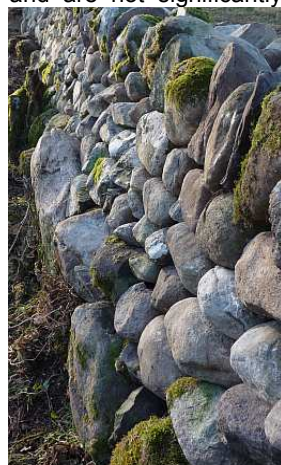
Fig.43. Original boulders left in situ and out of line, providing springboard for sheep
