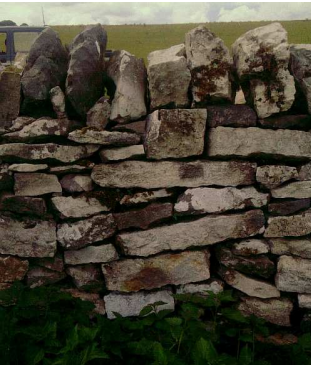
Fig.10. These two photos are taken close by in the same wall. The right hand photo is indicative of walls in the immediate area. This suggests that many of the through-stones were traced as building stones, in one short section (left)
