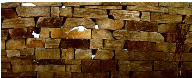
Fig.14. Relatively large gaps in sawn sandstone wall
