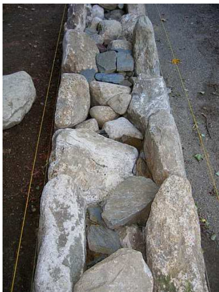
Fig.44. Inappropriate footing set on edge
