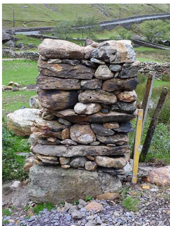
Fig.53. Poor ties and batter in wall end
