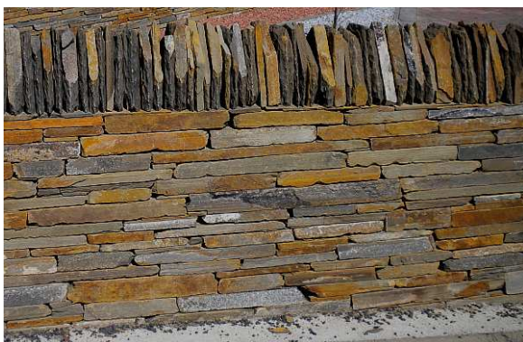
Fig.11. “Illusory” tracing, coal measures sandstone, Caithness
